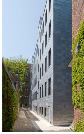
Twenty years ago, stucco was applied poorly to the side and rear elevations of this 40-unit apartment building near Harvard Square. The stucco eventually delaminated and began to fall off the building, after it had trapped moisture and had caused significant damage to the masonry bearing walls.
