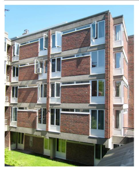
This project replaced 350 original steel windows with new aluminum windows, during a summer shutdown of an undergraduate dormitory built in 1968.
