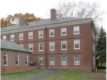
A fire wall divided this dormitory (built in 1923) into two, and each side had only one egress stair supplemented by a collection of fire escapes and ladders.
