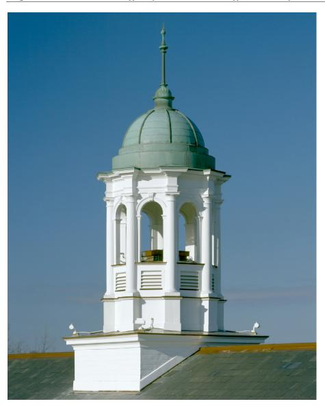
We designed and oversaw the restoration of this historic, 100-year old cupola (originally designed by McKim, Mead and White). Paint was stripped to the bare wood, extensive carpentry repairs were made, and pre-patinated copper was used for the dome sections in order to match the patina of the existing decorative ribs and spire which remained.
